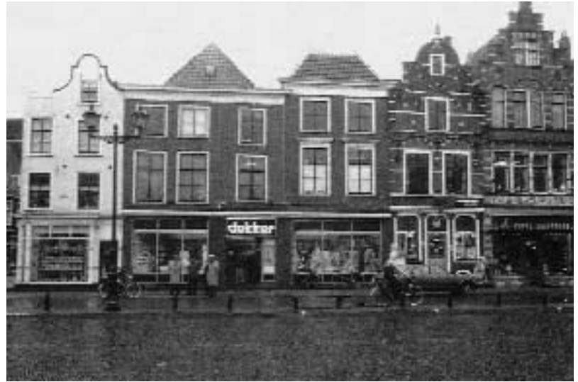
Figure 5.15 Paved square, Delft
